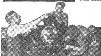
Students wiring and checking ignition on one of the late type Radial Aircraft Engines in our aviation department
